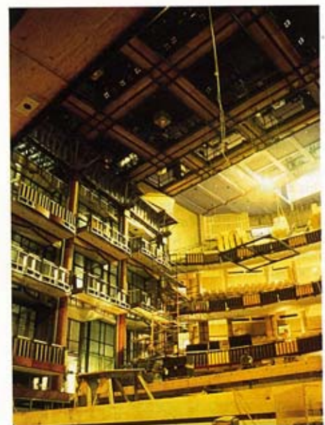
Cerritos: The auditorium taken from the orchestra pit showing lighting bridges and 'hinged' auditorium towers.
